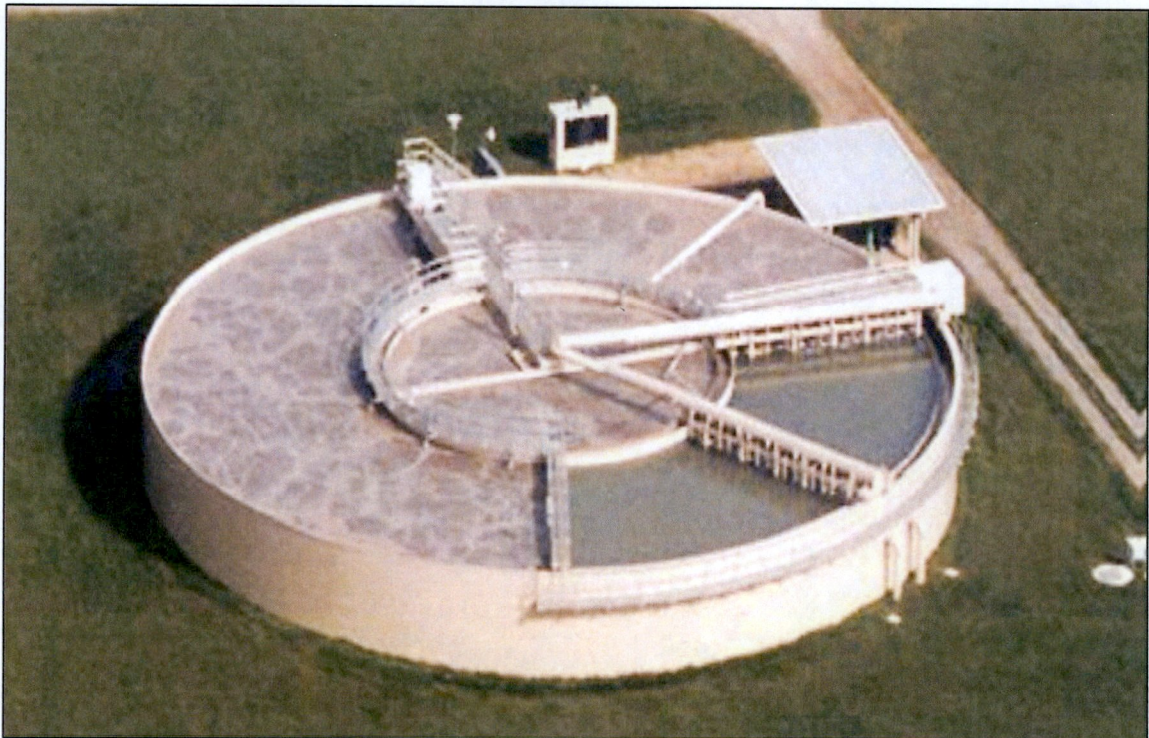
Figure 5.0: Davco Field-Erected System Example, 1MG Dual-Path Process
