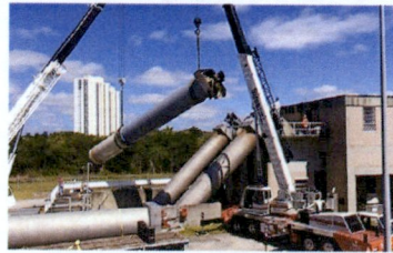
Inspect, repair or replace screw pumps
